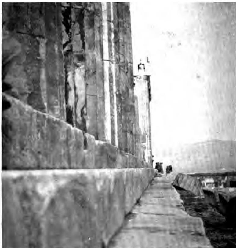
THE PARTHENON, STYLOBATE SHOWING CURVATURE Athens
